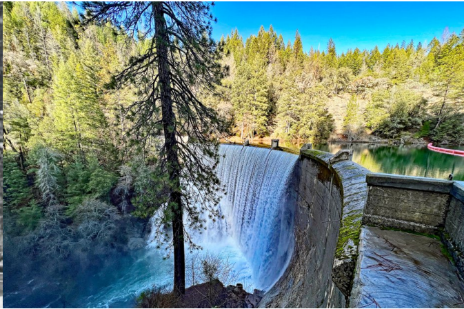
Deer Creek Reservoir Dam in January 2023
