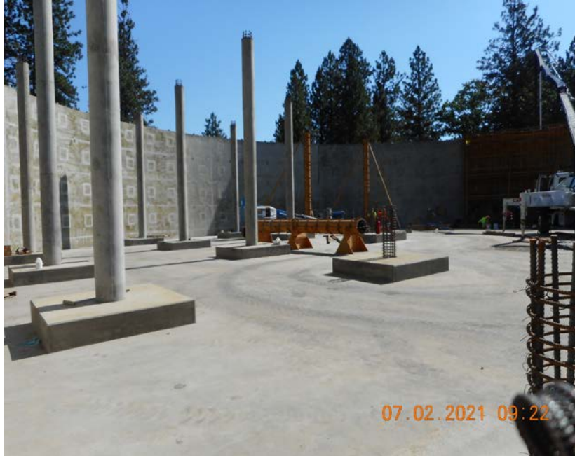
Alta Sierra Tank Site Construction
