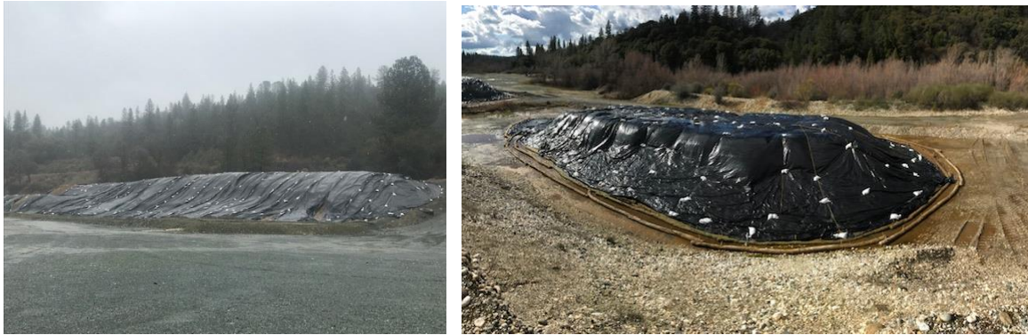
Sediment Stockpile SWPPP
