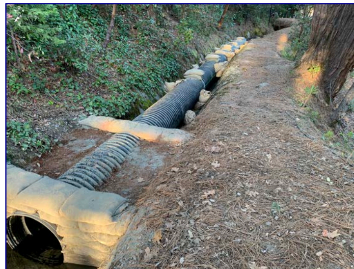
Snow Mountain Canal Encasement Canal Maintenance Crew
