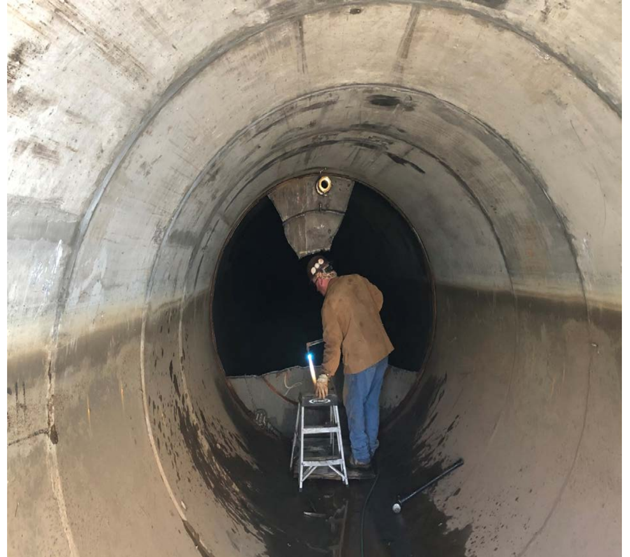
Removal of steel bulk head on April 9, 2021
