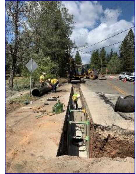
Ridge Road Pipeline Replacement Construction Crew
