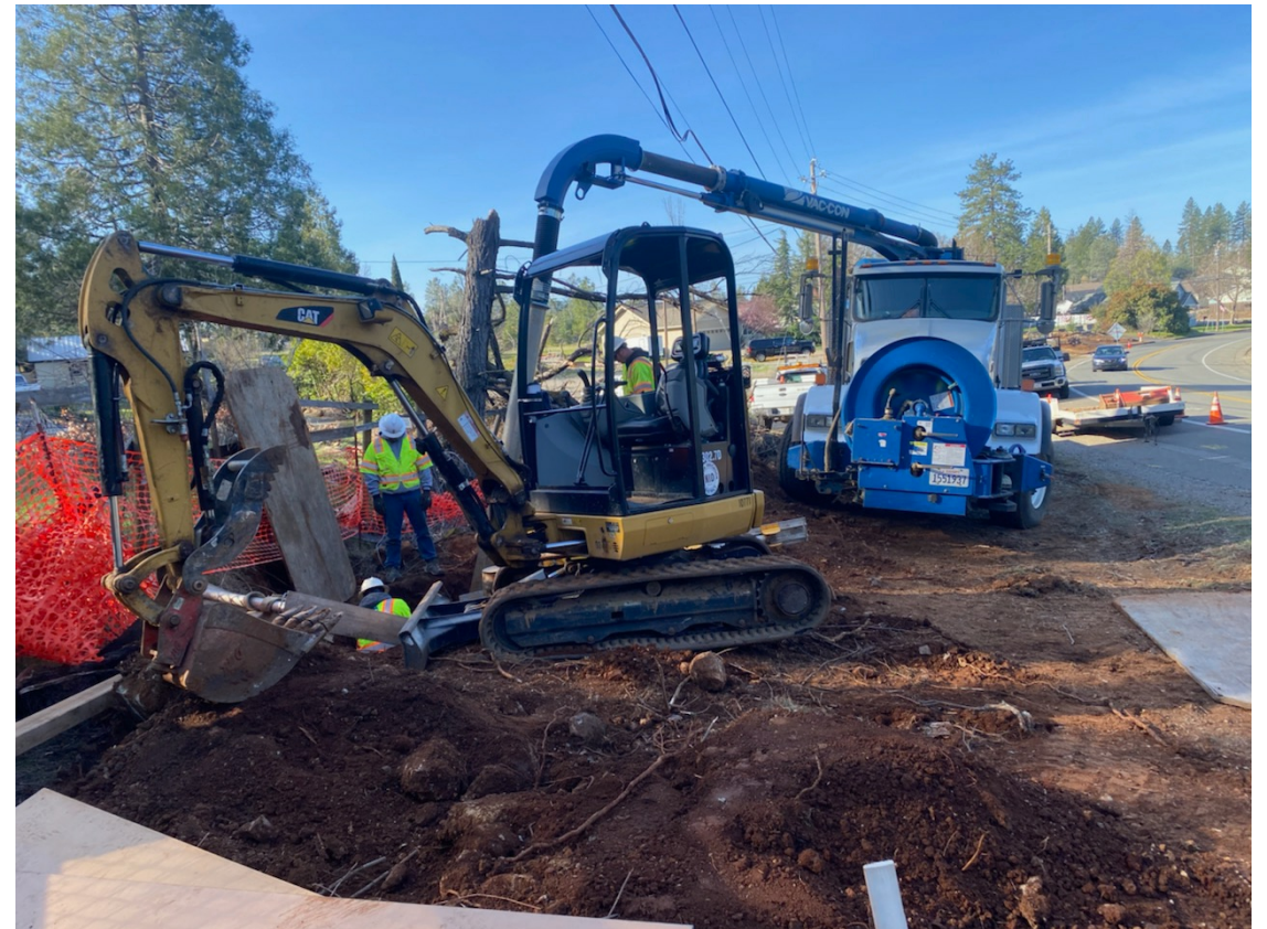
Up grading the transmission main line on Ridge Road, upsizing 10 inch pipe to 20 inch pipe
