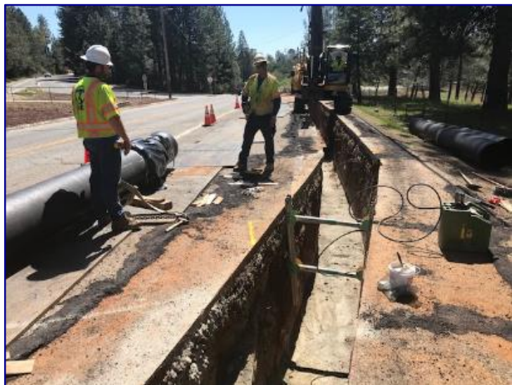
Ridge Road Pipeline Replacement Construction Crew
