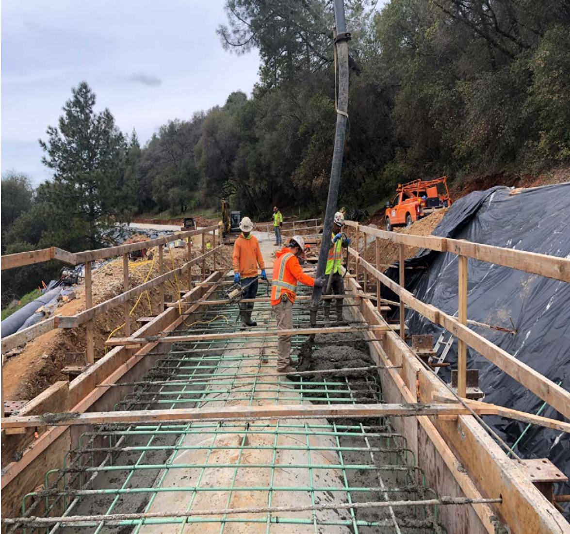
Crews encasing a section of pipeline, March 17, 2021
